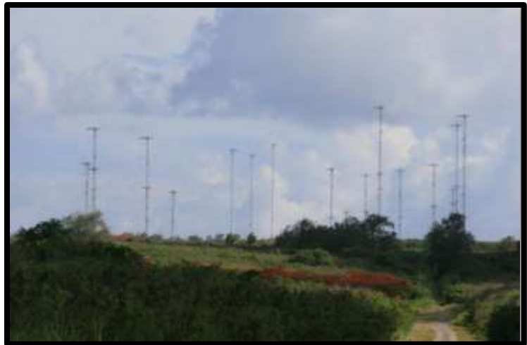
Photo 3.6-1. International Broadcasting Bureau Antenna Array
