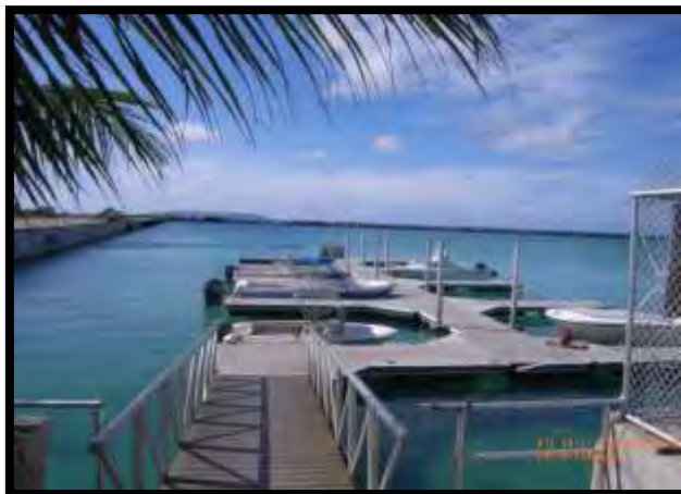
Photo 3.8-20. Mooring Slips at Tinian Small Boat Dock
