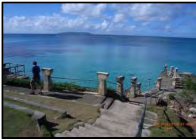
Photo 3.8-17. Unai Taga Stairway to the Beach and Overlook Platform with Aguijan Island in the Distance
