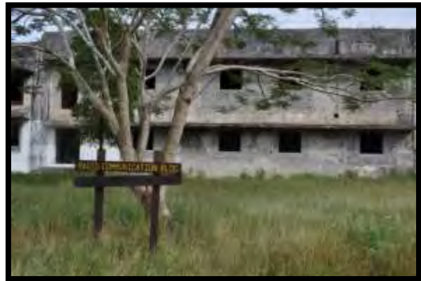
Photo 3.8-7. Japanese Radio Communications Building along Broadway Avenue
